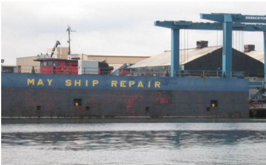
Mariners Harbor, Bulkhead and Piers at May Ship Repair 06.27.2014
